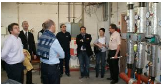
Visite sur site – Village N°1 Reine Fabiola
